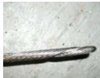
Non-approved metal cable and metal unraveling.
