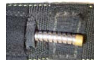
Housing out of place, tacking missing.
